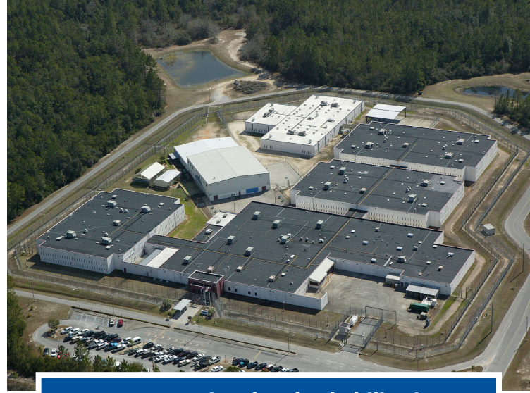
Bay Correctional and Rehabilitation Facility, Florida
