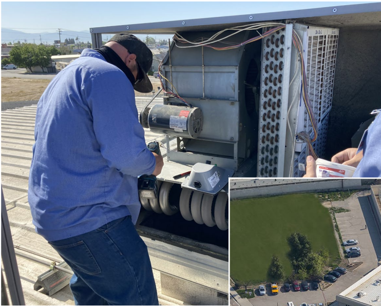
Bi-Polar Ionization units being installed at the Mesa Verde Processing Center
